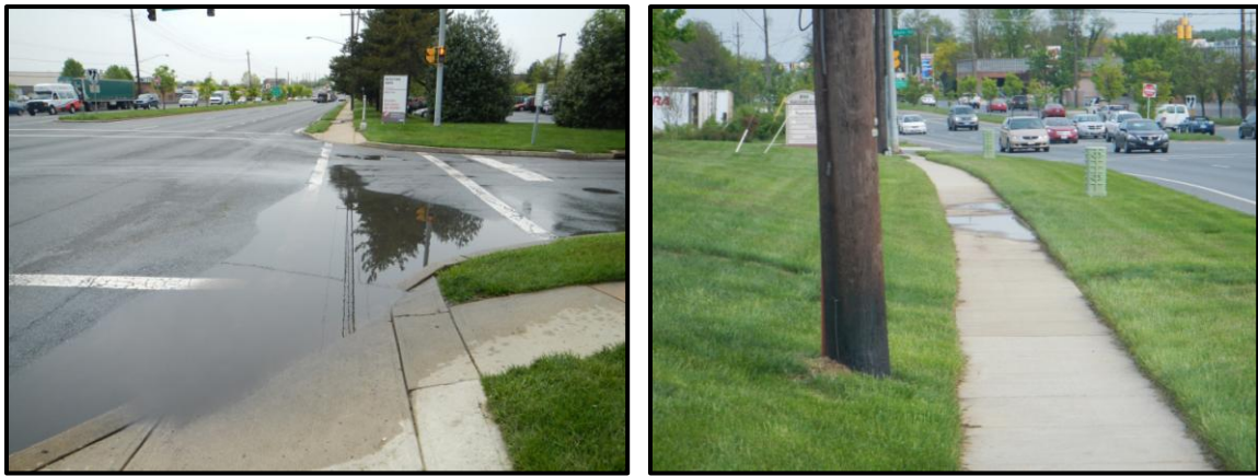
Left: Ponding near the intersection of E Gude Drive at Calhoun Drive. Right: Water ponds along the sidewalk between the MCCH and Dover Road.
