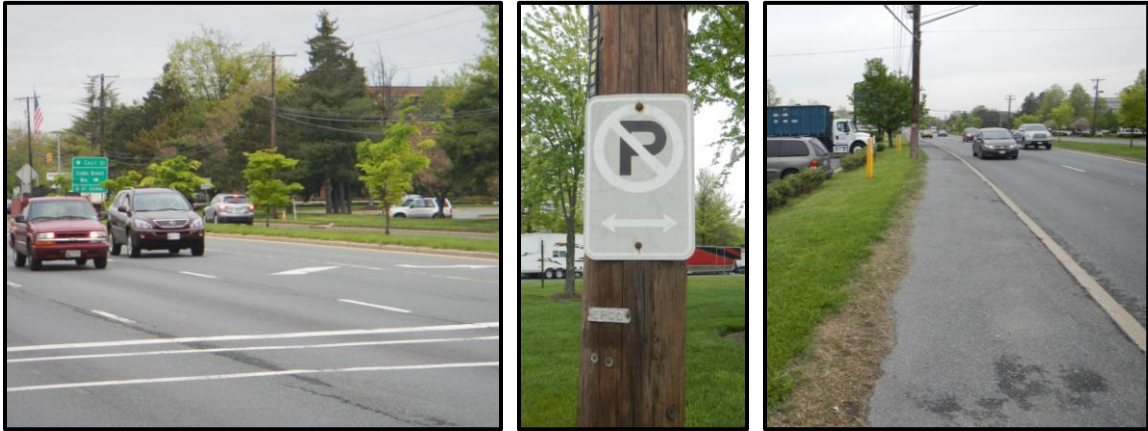
Left: Lane drop pavement marking arrows near Calhoun Drive are faded. Center: Sign is faded and is non-retroreflective. Right: Overgrown vegetation on the Millennium Trail reduces the effective trail width.
