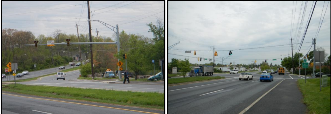
Left: Pedestrian crossing at the modified HAWK signal without activation and outside of the crosswalk. Right: Lane configurations are not supported by lane use signs on the eastbound approach at Dover Road.
