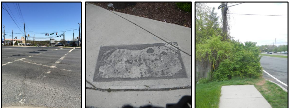
Left: Crosswalk at E Gude Drive at Southlawn Lane is faded. Center: Missing Detectable Warning Surface near Liberty Gas Station. Right: Sidewalk ends prior to the MCCH driveway.
